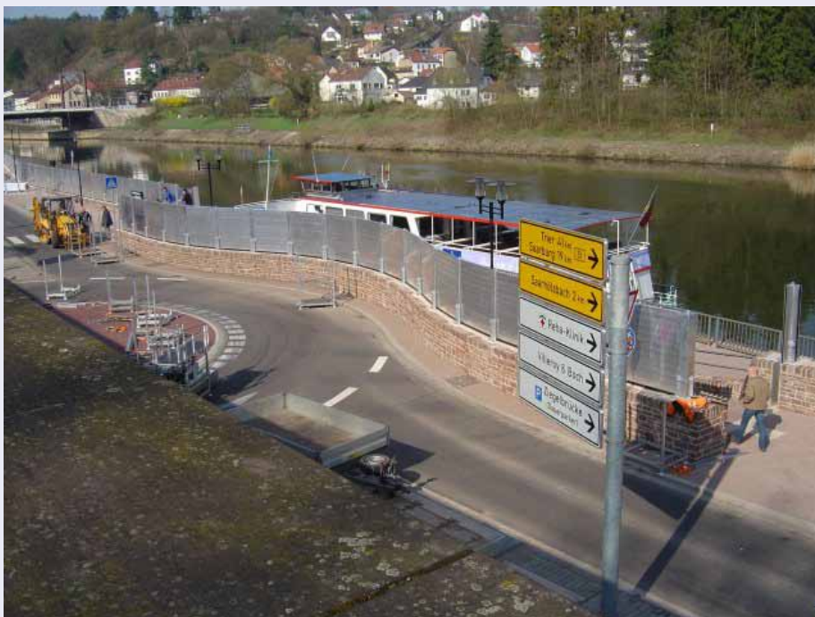
Because it is not possible to provide rivers with permanent dykes over their whole length, mobile barrier systems are also in demand. For some time now the sandbag has faced competition from devices such as tubular systems, interlocking mesh modules and mobile walls.
