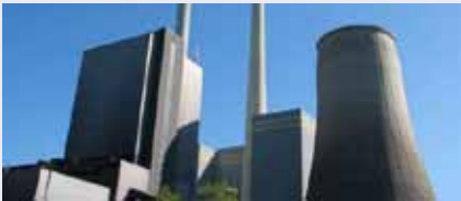
Trials of the first 700 degree power station are to start in 2014.
